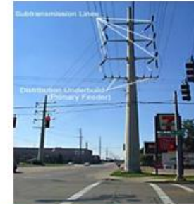
Primary Distribution Facilities
